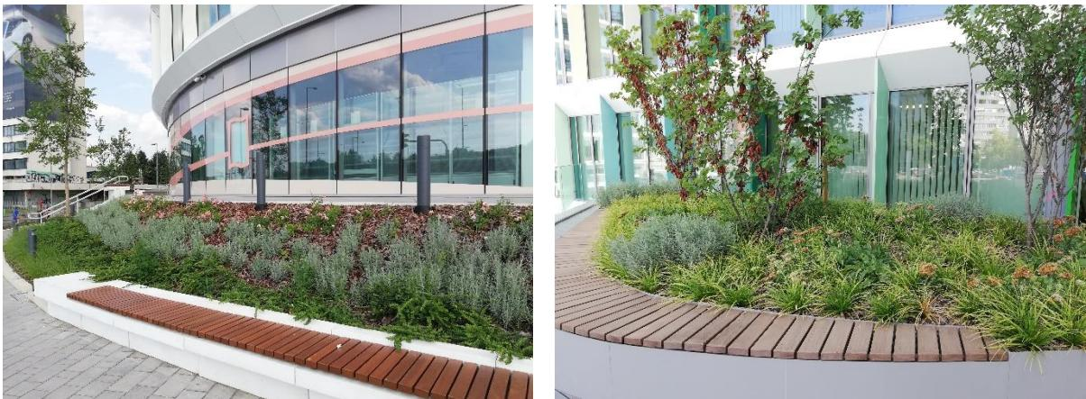
The principle of generous arches played an important role during the formation of the borders between green and paved areas on the outer side of the building. As the level difference is growing along the Koszorúslány Street, retaining wall system was constructed with slopes between and in front of them. The strips, which run almost parallel are decorated with ornamental grasses, flowering perennials and evergreens.
