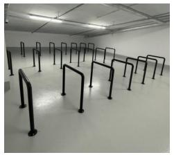
On level P1, there is 131 m2 of bicycle storage in 2 rooms, one of which has a simple storage facility, while the primary storage room has a bicycle storage area with a double-decker design. The bicycle and pedestrian access to the storage area is separated from the car storage area, with a separate entrance and exit to Szigony Street, and therefore cycling is not permitted in the rest of the garage.
